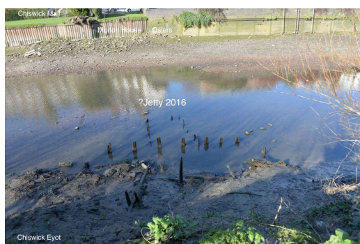
Timber structure in the Thames, from the Eyot looking north, 2016
