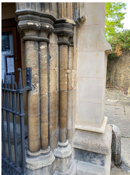
North porch showing old and new stonework Photograph: Francis Ames-Lewis
