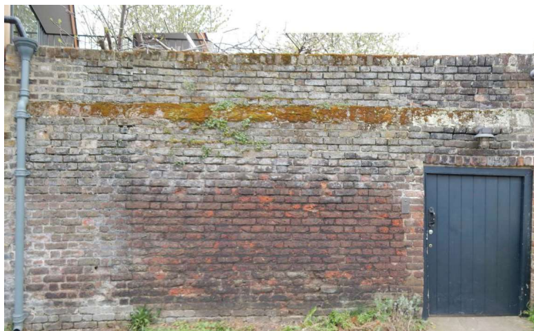
Boundary wall along Netheravon Road South at Morton House
